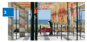
Joists are hung by one end from a ledger and then rotated into position at the opposite end by a single worker.
